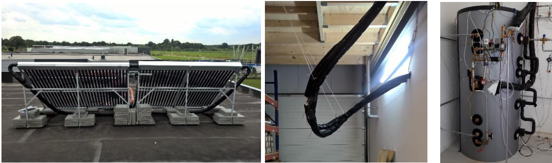
Fig. 2: Images of direct solar system with TDBV; collector array (left), adjustable negative loop (middle) and the storage tank (right) with TDBV installed at 0.5 relative height, and thermostat valve at 0.8 relative height
